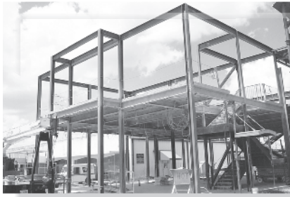
Typical steel framework.
