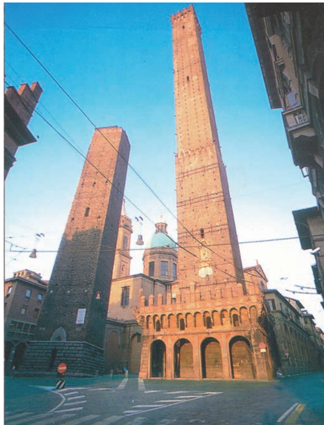
FIGURE 1.4 Tilting of Garisenda Tower (left) and Asinelli Tower (right) in Bologna, Italy (Courtesy of Braja M. Das, Henderson, Nevada)
